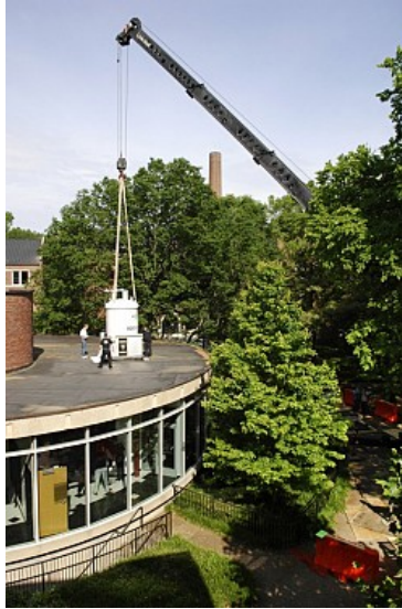
The massive new magnet was lowered by crane, with just four inches of clearance. (photo by Anne Rayner)
